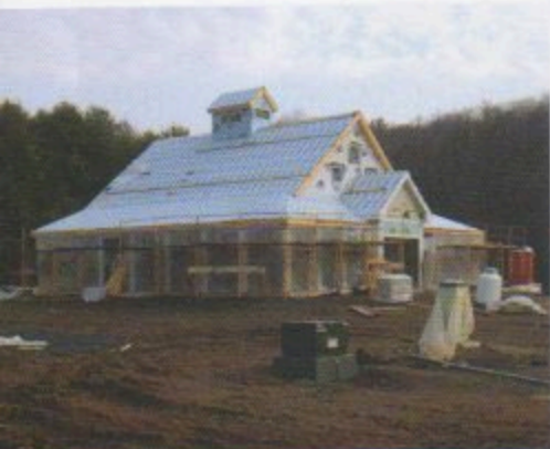
Work in progress on the Maurice D. Hinchey Catskill Interpretive Center.
